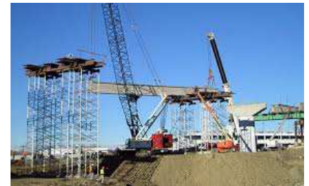
Erection Tower—Lifting Analysis
